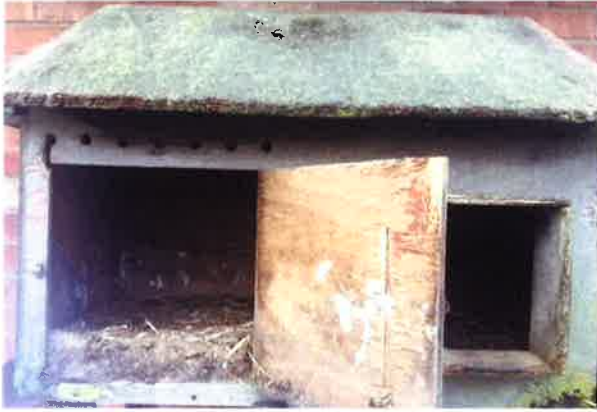
Horbling Pumping Station (8): Before
