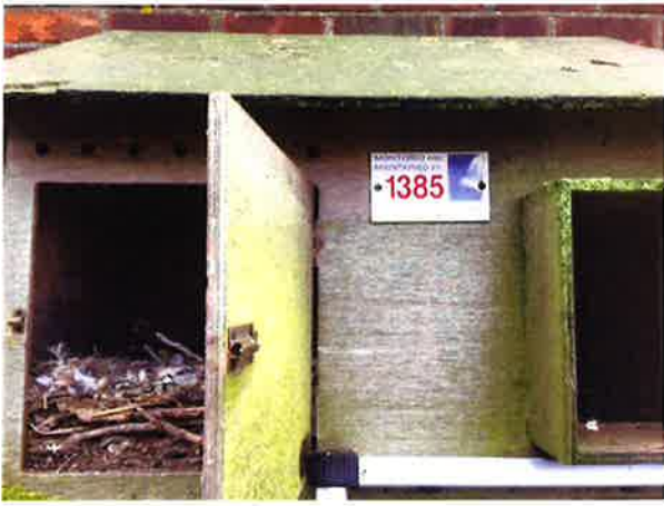
Ewerby Pumping Station (4): Before
