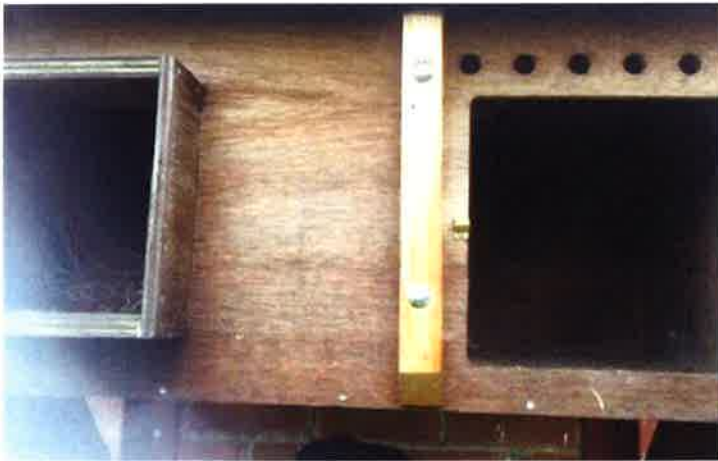
Helpringham Pumping Station (6): Before
