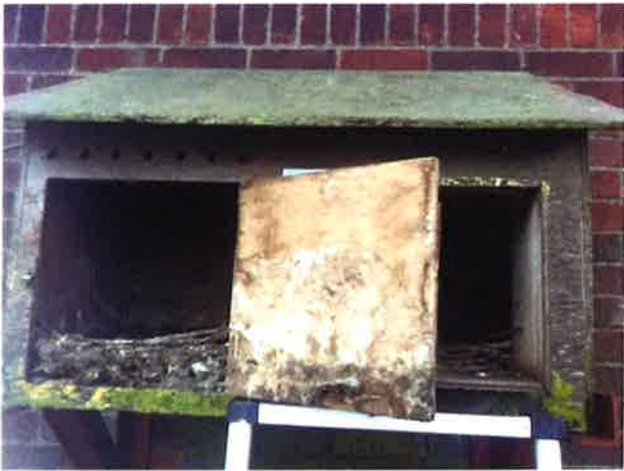
South Kyme Pumping Station (2): Before
