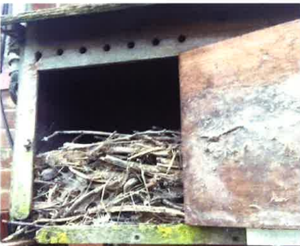
Dowsby Lode Pumping Station (12): Before
