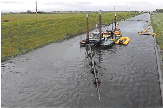
10" Cutter Suction Dredger 'Phoenix'
