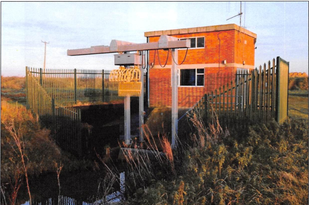
Horbling Fen Pump Station (for comparison)
