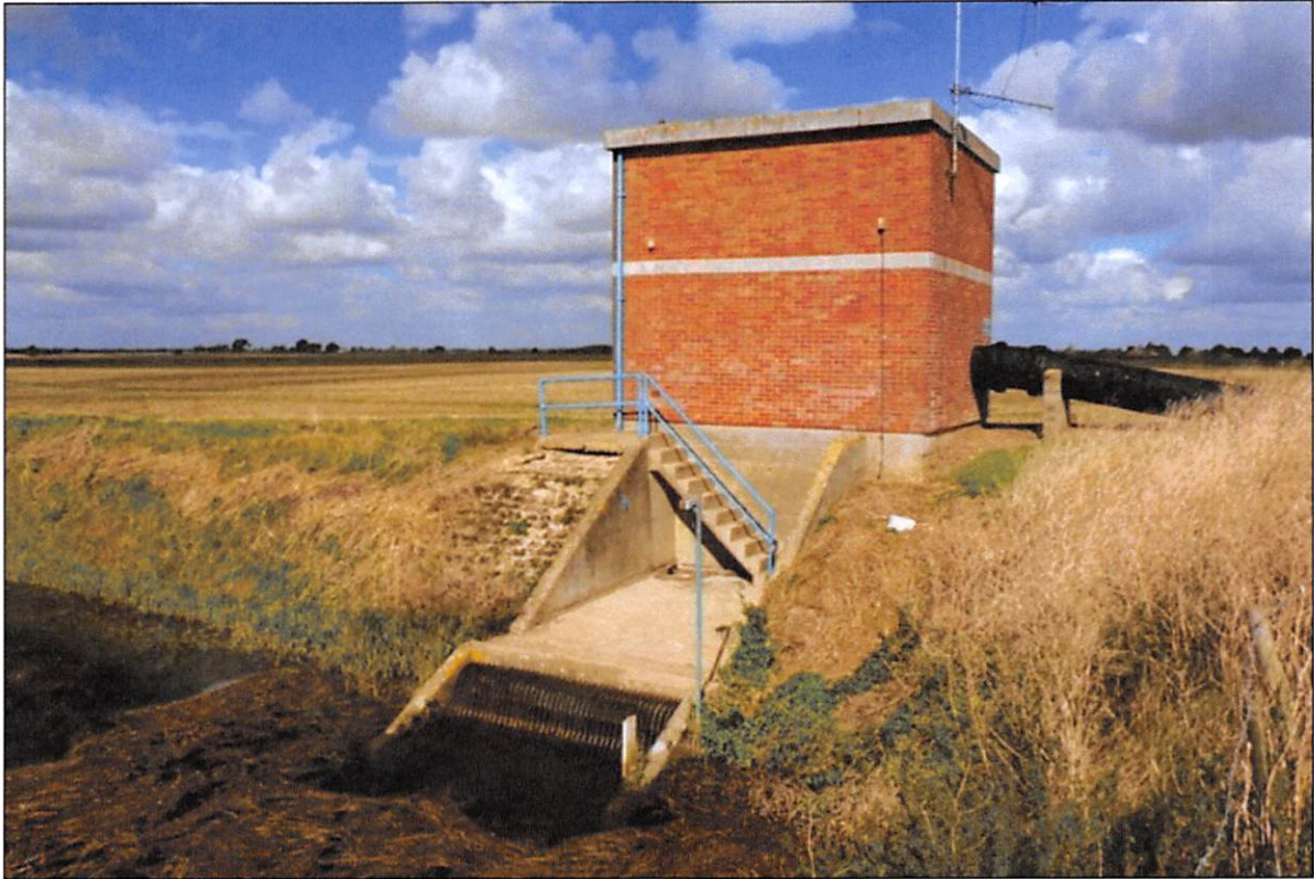
Sempringham Fen Pump Station
