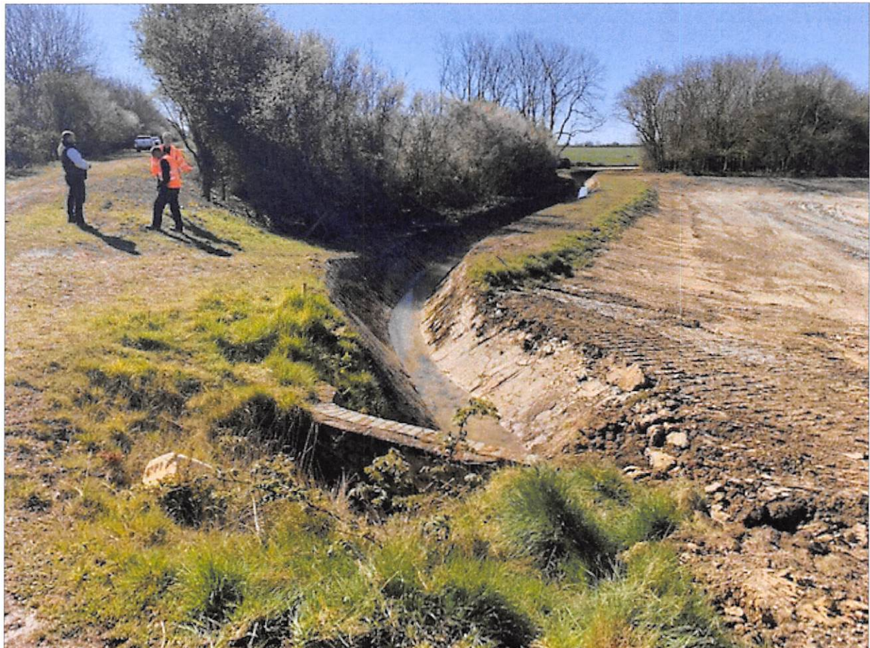
Holland Road Farm works to replace the spillway have now been completed.
