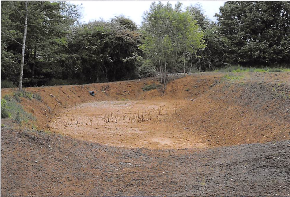
Enlarged pond with swale & outfall pipe
