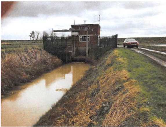
General view of pumping station end
