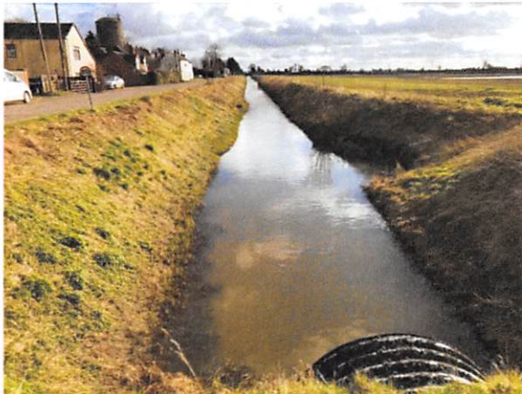
General view SE from Holland Fen
