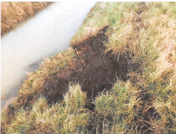
Bank slip near field boundary ditch
