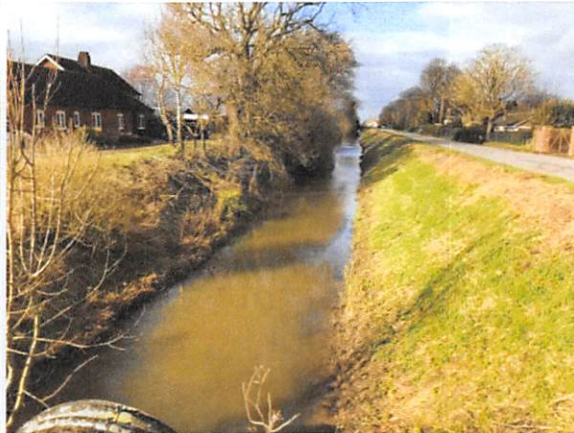
General view NW from Holland Fen (note small ash trees at the culvert)
