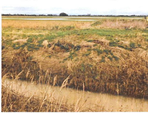
Old brickwork on north bank
