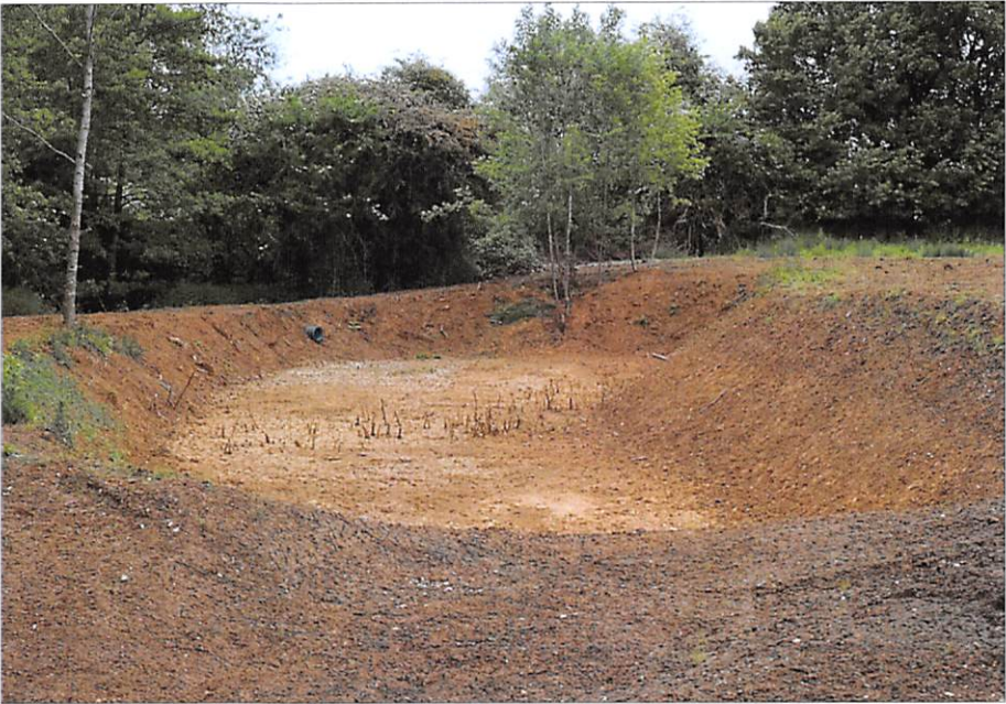
Enlarged pond with swale & outfall pipe
