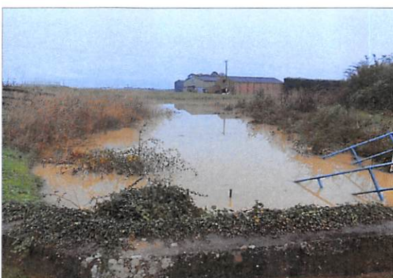
Helpringham Fen PS and South Forty Foot Drain outfall
