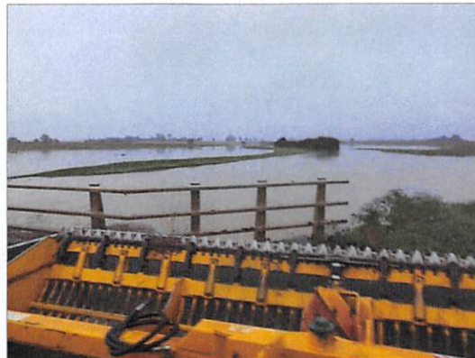
Flooding EA North Beck Burton Bridge Burton Pedwardine
