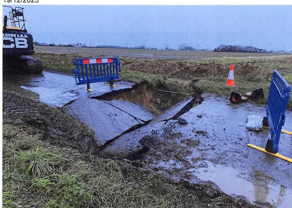
This is how the operatives found the site when they arrived in the morning. It can be seen that despite the machine being parked on the road, a vehicle has driven past it and maybe is the cause of the failure. This photograph was shared with LCC and stated to them that the decision to remove the culvert was not just due to conveyance of flows but also from a Health and Safety viewpoint, due to the failure of the road this was evidently the right decision.
