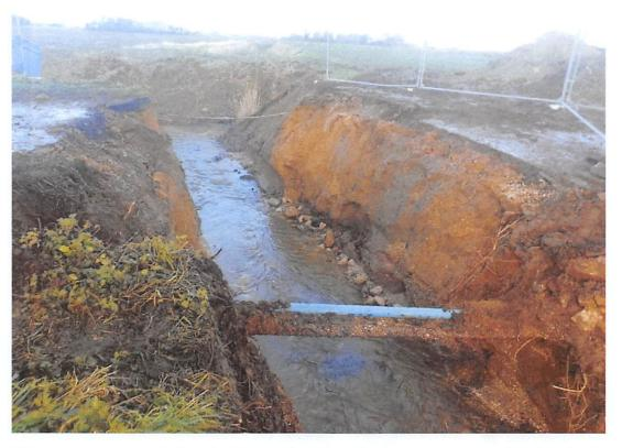
After culvert removed, showing flows reinstated. Harris fencing shown hired by the Board.
