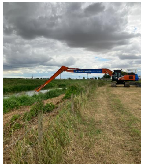
Channel desilting work on the Lower Barlings Eau.
