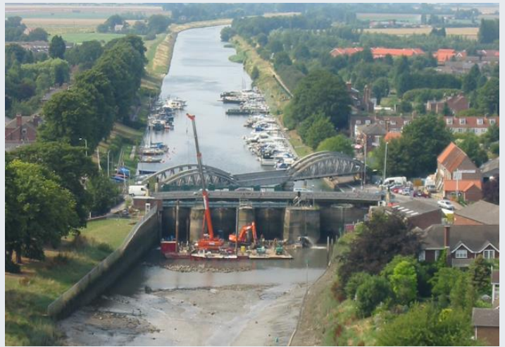
Previous refurbishment works carried out at Grand Sluice in 2006.
