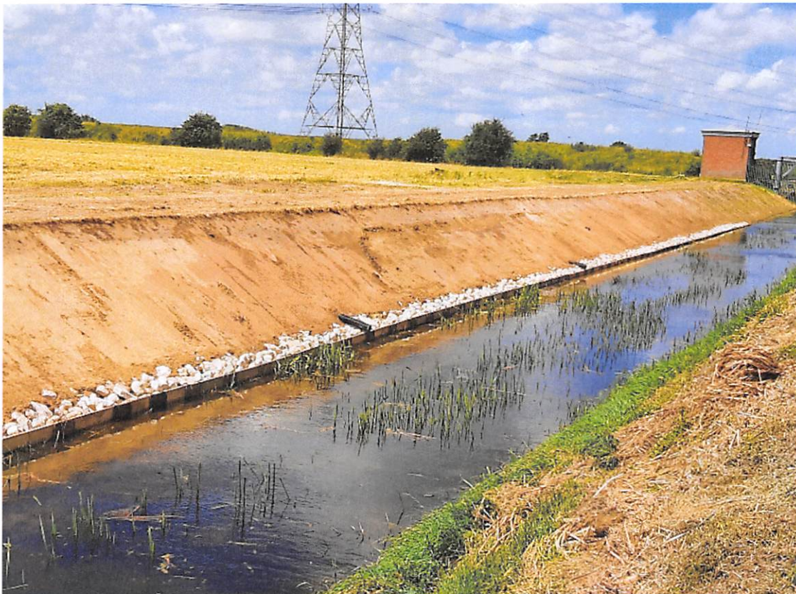
Slip Repair at Bicker Fen
