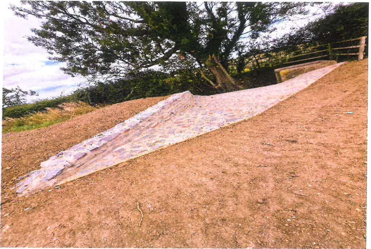
Completed spillway
